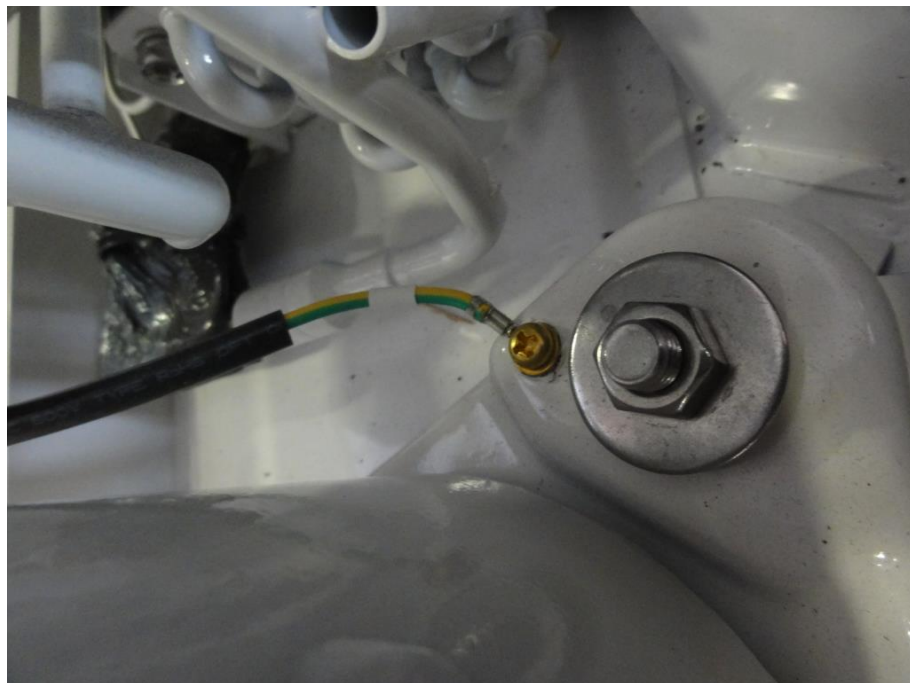
Earthing screw for compressor
